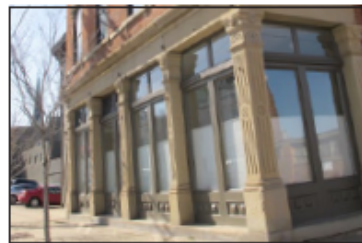
An example of a shopfront with formal pilastered bays
