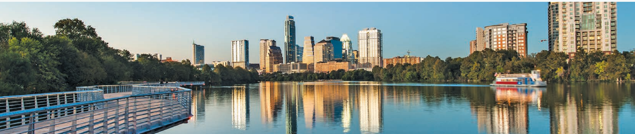
Boardwalk on Lady Bird Lake by Limbacher & Godfrey Architects
